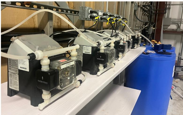
chemical being used, the diaphragm pumps were having reliability issues, including diaphragm failure, loss of prime, and chemical leaks.
